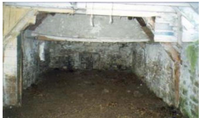
This byre, in a poor state of repair, was once a dwelling as can be seen by the fireplace at the gable end. It is of architectural interest because it contains crucks, an early form of roof supports built into the walls.
