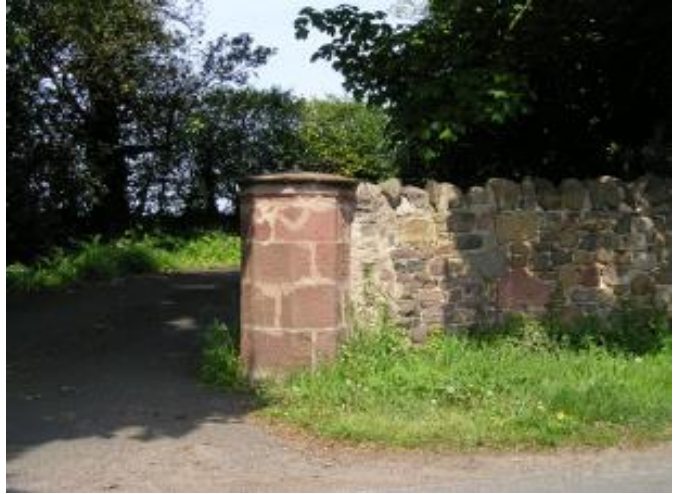
Well-restored gateposts can enhance the visual impact of farms. The mortar pointing could have been more carefully finished on this example.
